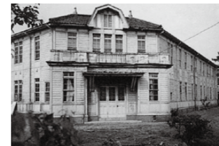
経済学部校舎(昭和45年当時) School Building of the Faculty of Economics (1970)
