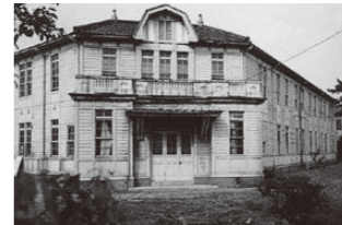
経済学部校舎(昭和45年当時) School Building of the Faculty of Economics (1970)
