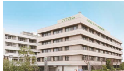
みどり市民病院外観 Nagoya City University Midori Municipal Hospital
